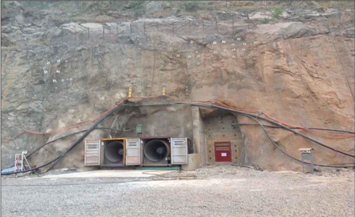
Figure 16-18: Akoti 2x315kw Exhaust Swedvent Fans
