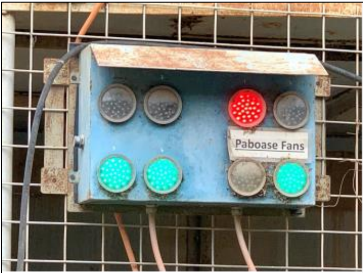
Figure 18-21: Primary Fans Indicator Lights
