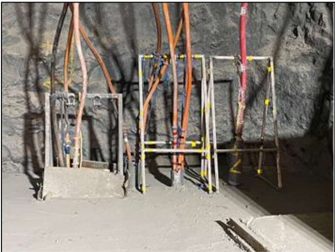
Figure 18-19: HV Cables through Service Holes at Suraw
